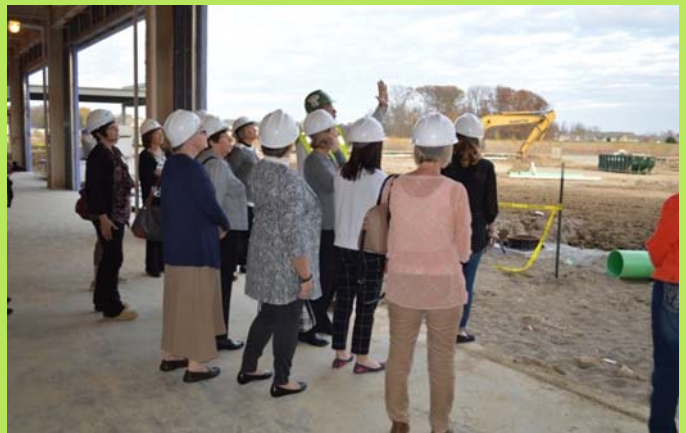
The committee ended the year with a construction tour of the new Medical Center.
